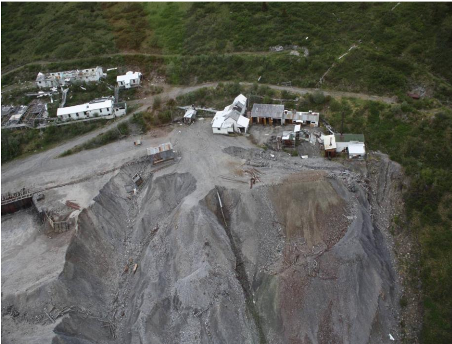
4. Keno 700 before the hazard reduction work.
